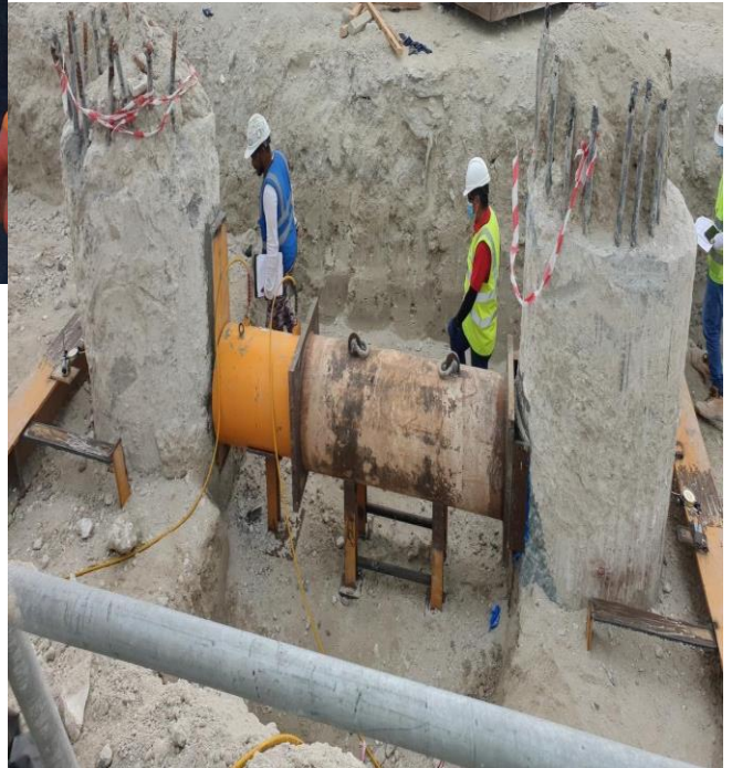
Lateral Pile Load Test
